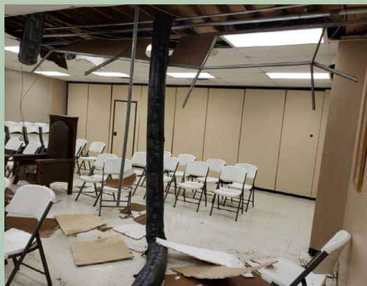
Outside, the roof has been damaged and the ceiling collapsed inside the hall, leaving a lot of rebuilding to be done and debris to be cleared away.
